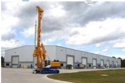
BAUER Manufacturing Inc. Conroe, Texas, USA
